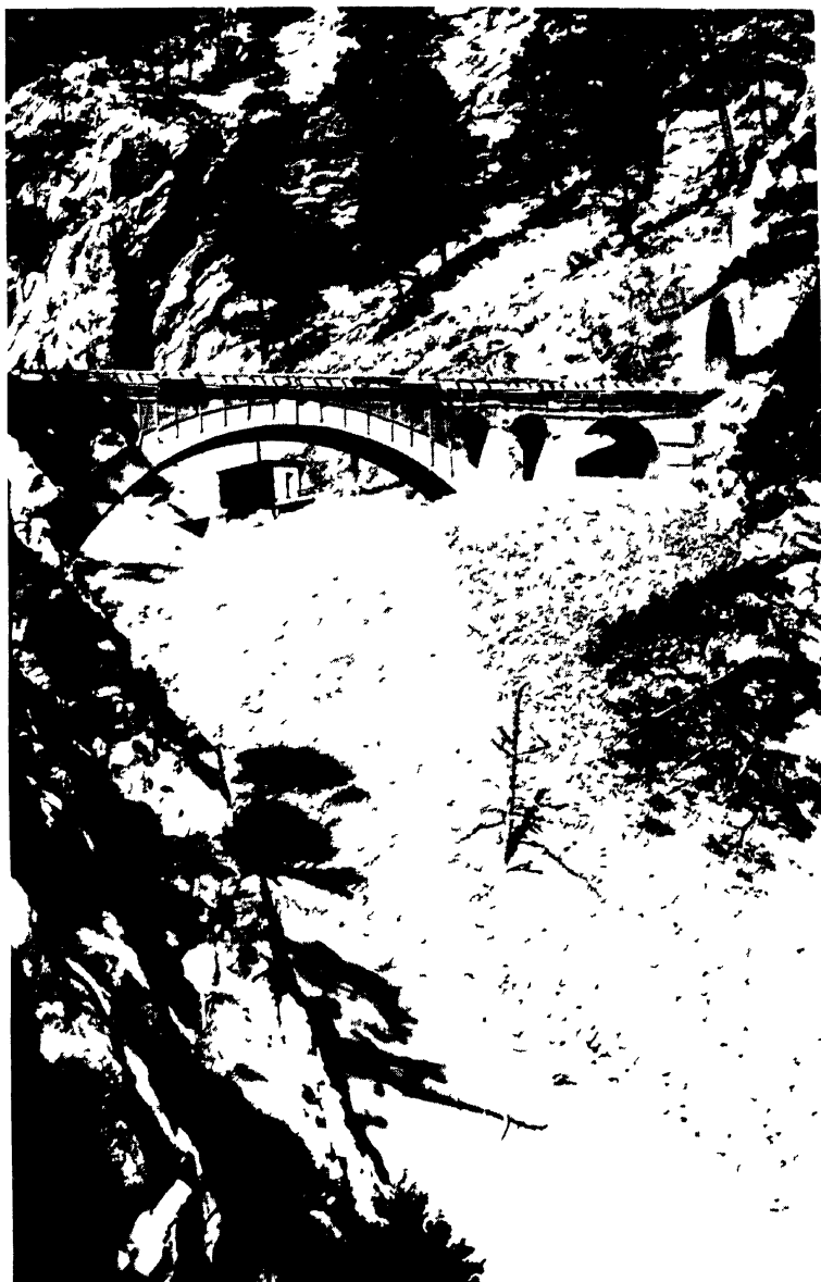
THIRTY METRE CONCRETE ARCH BETWEEN TUNNELS, BAGHDAD RAILWAY
