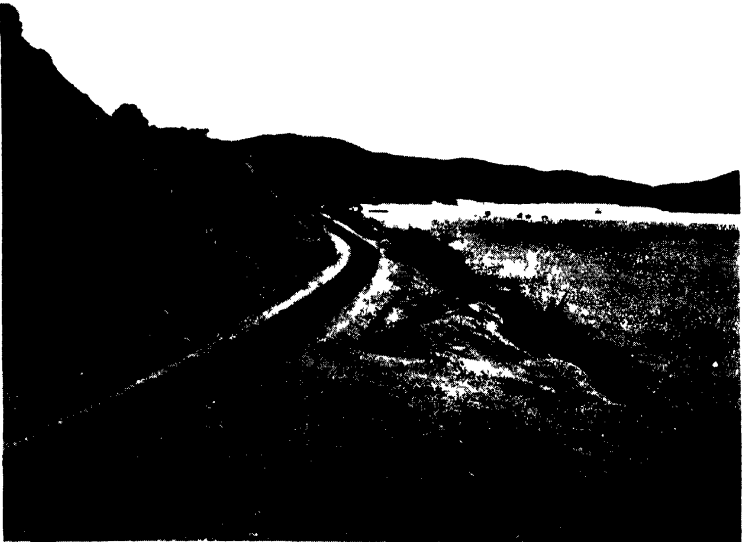
RAILWAY CONSTRUCTION ALONG THE PI HO RIVER
